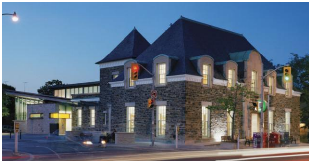
Runnymede Branch with new extension
