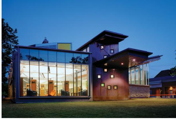
The new extension showing the exterior copper wall
