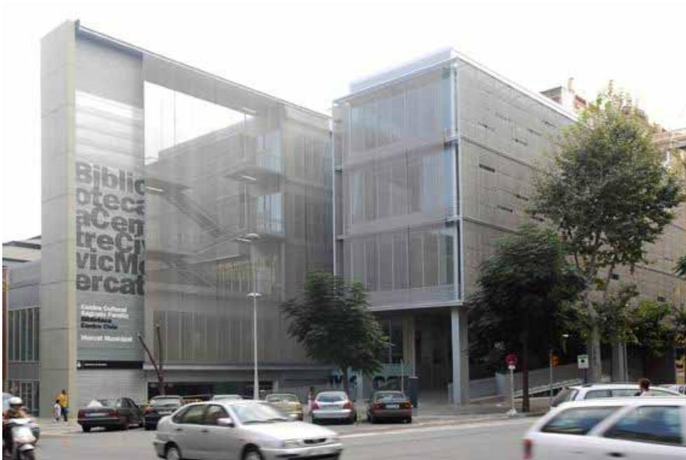
In order to describe the external appearance of the **Biblioteca Sagrada Família**<sup>vii</sup>, in Barcelona (opened in 2007) the architect Manuel Ruisanchez<sup>viii</sup> explains “A perforated aluminium filter acts as an opaque surface that reflects the sun during the day and creates the illusion of the awakening of a lamp during the evening and at night”<sup>ix</sup>.
