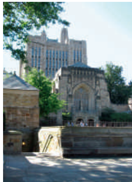
1. Sterling Memorial Library at Yale University. The main stack tower is one of the experimental sites for the project.
