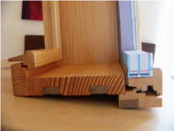
3. Presentation of a prototype as basis for discussion at the 3ENCULT window workshop – outer wing can keep original single glazing (source PHC/ANDRE).
