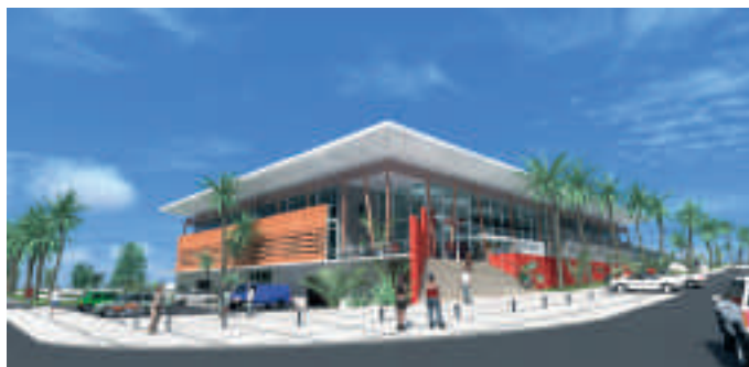
2. West side. View on the entrance hall and public area of the Territorial Archives.
