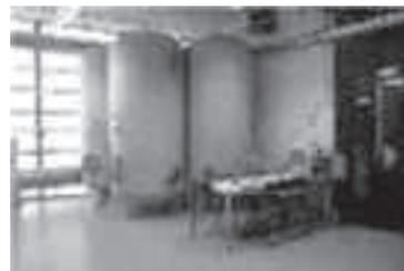
3) A treatment unit with three rigid containers A, B, C with a volume of 1x25m<sup>3</sup> (B) and 2x35m<sup>3</sup> (A, C).
