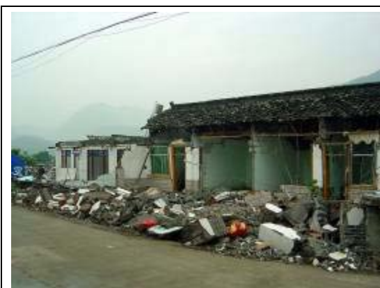
Pic31 After the earthquake
