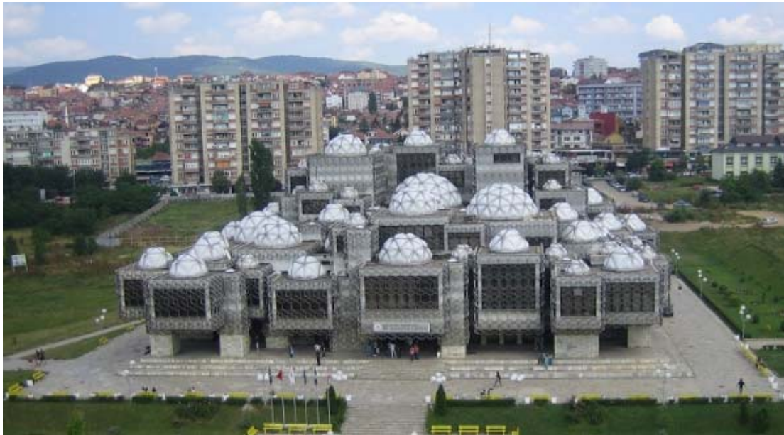
Photo 1: The building of the National and University Library of Kosova
