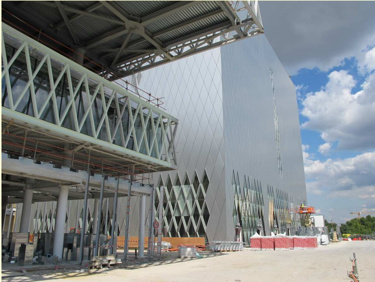
The new building in completion
